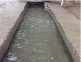
Plate 4: Lined surface water channel for Irrigation Purpose near Hanzel Bala Village
