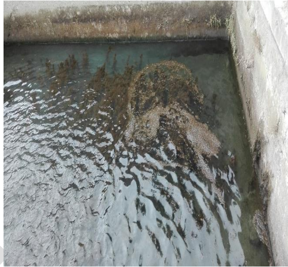
Algal growth in storage tanks of Barmus Water Supply Complex
