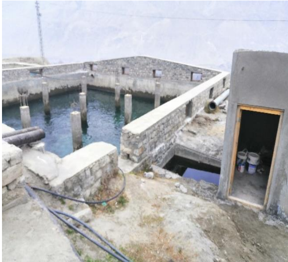
Storage of paints and other chemicals adjacent to water tank, possible source of chemical contamination.
