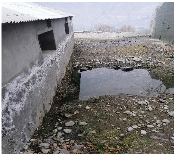
Seepage /infiltration of overflowing water into water storage tank, possible source of contamination.
