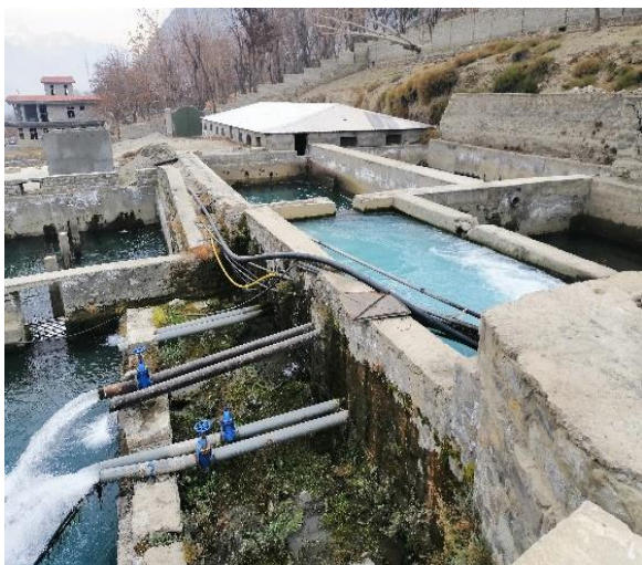
Poor/rudimentary infrastructure of water supply system, as overflowing water from upper tank gets its way into next tank accompanied with pollutants. Sanitary condition is very poor and algal growth can be seen.
