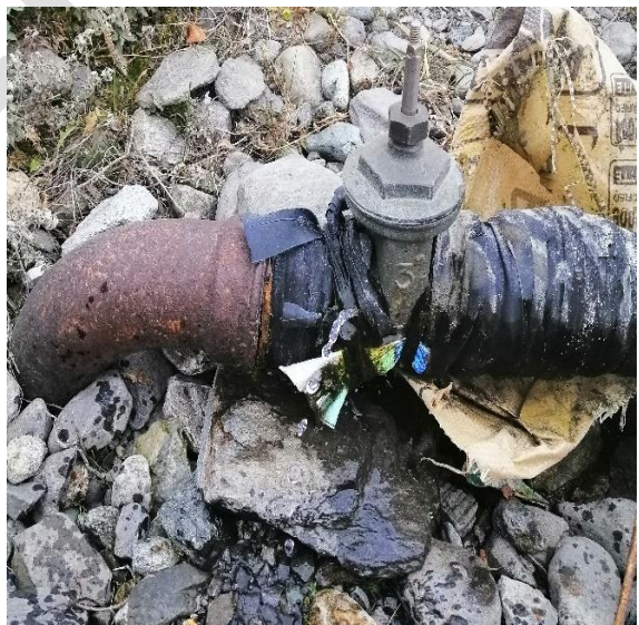
Broken Values and pipes exposed to ingress of pollutants in water.
