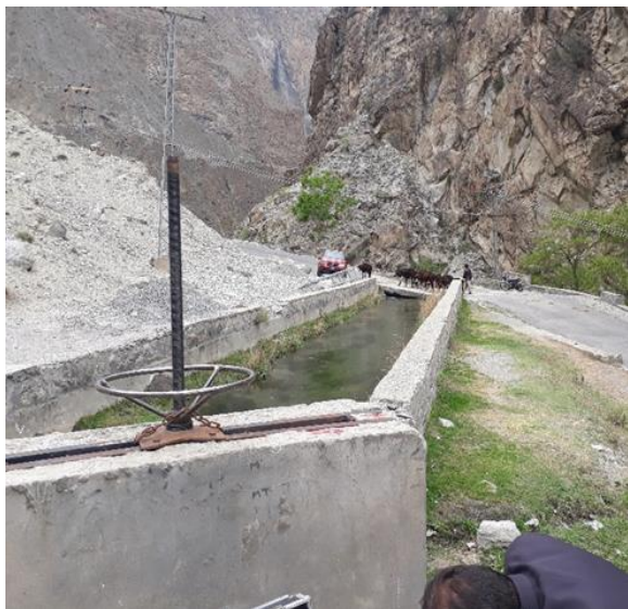
Inferior design of open intake system exposed to contamination.
