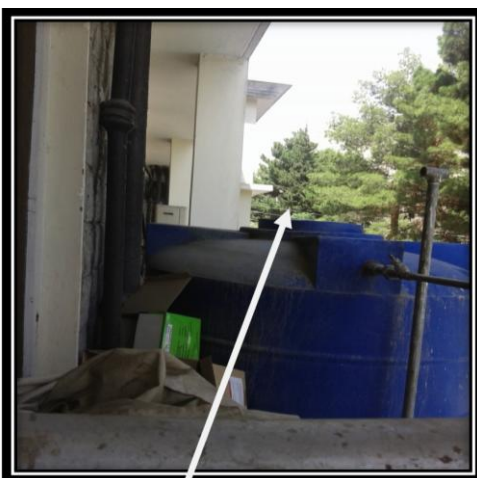
Fig. 4. Overhead tank without cover at DHQ Hospital.
