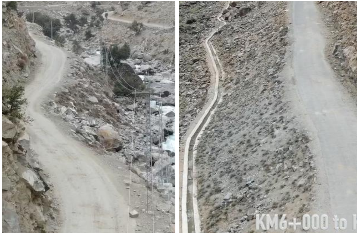
Figure 7-2: Views of electric poles and water channel to be relocated falling in RoW
