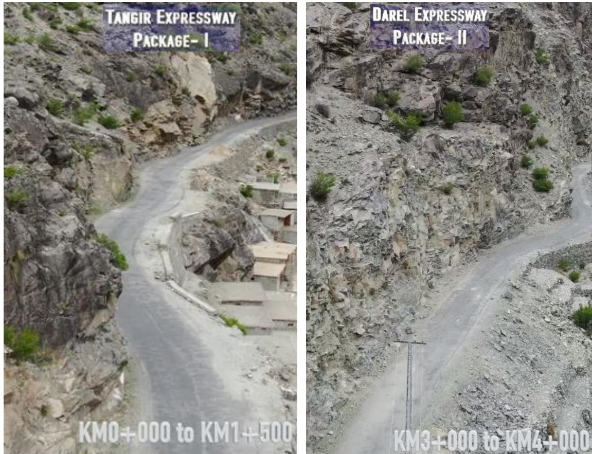
Figure 7-4: Blasting will be required to remove such hard rocks while constructing Tangir and Darel Expressways.
