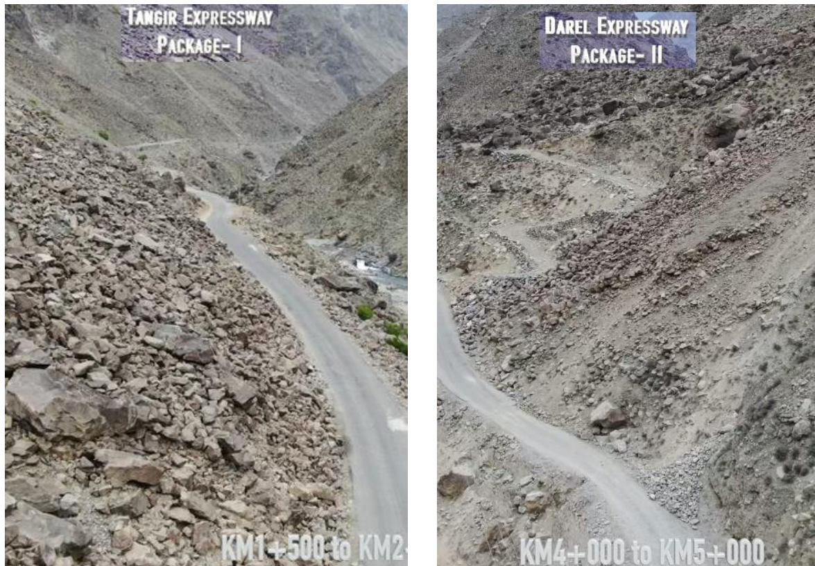
Figure 7-3: Views of unconsolidated materials, where land sliding may trigger during construction.
